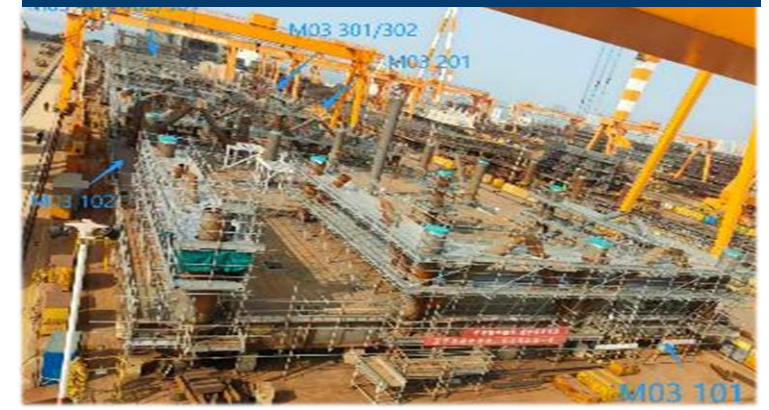
Module structural assembly ongoing
